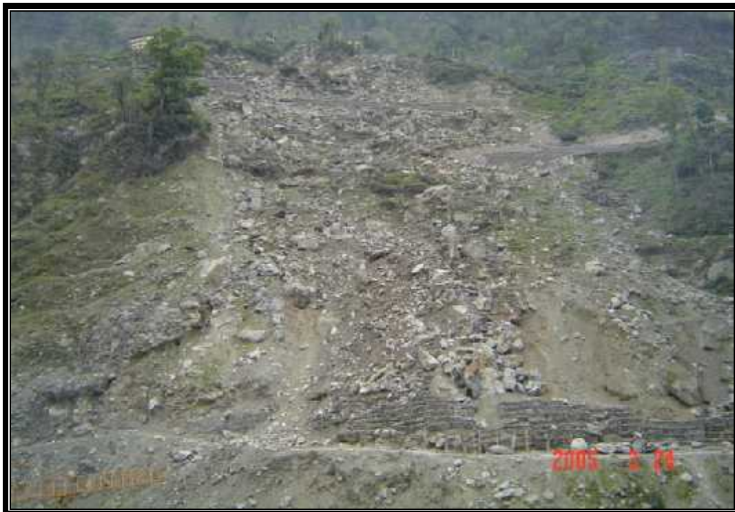
GABIONS OVER UNSTABLE SLOPE, DAM SITE, NHPC STAGE V, SOUTH SIKKIM
