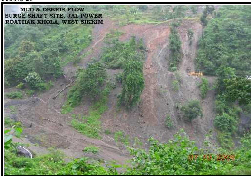
MUD & DEBRIS FLOW, SURGE SHAFT SITE, JAL POWER, ROATHAK KHOLA, WEST SIKKIM
