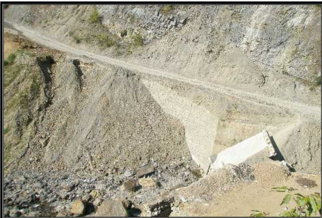
COLLAPSED BRIDGE ON NAMCHI - BUL ROAD, NEAR SALEBONG, SOUTH SIKKIM
