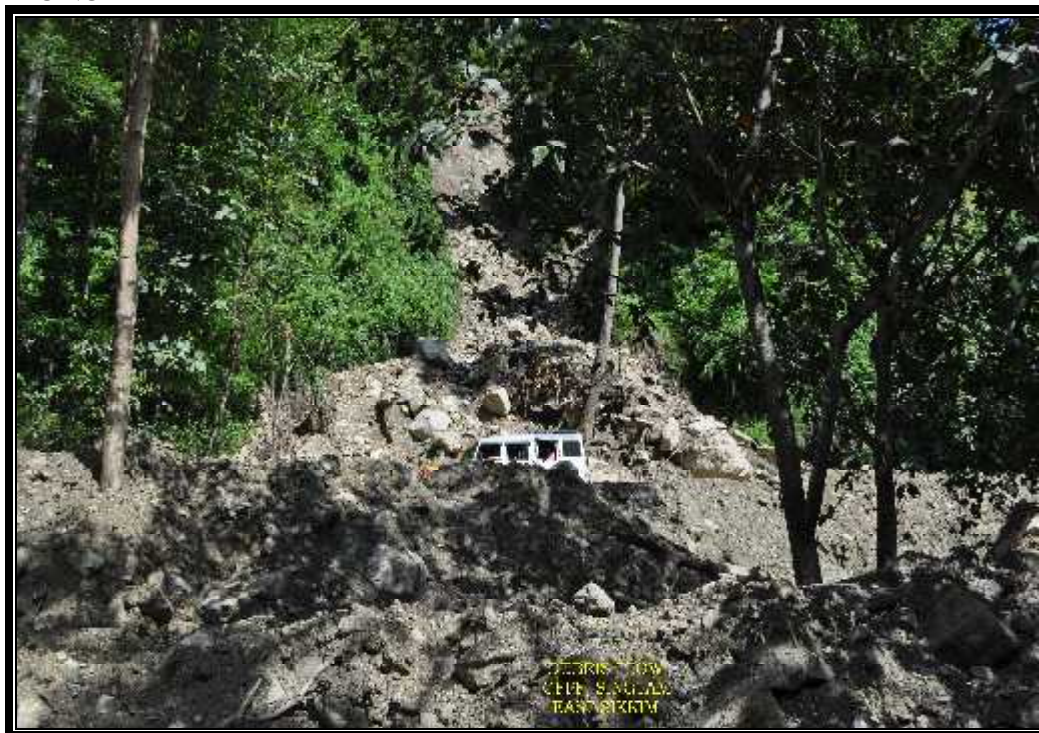
DEBRIS FLOW –CHISO PANI LANDSLIDE ALONG NH 31 A, NEAR SINGTAM, EAST SIKKIM
