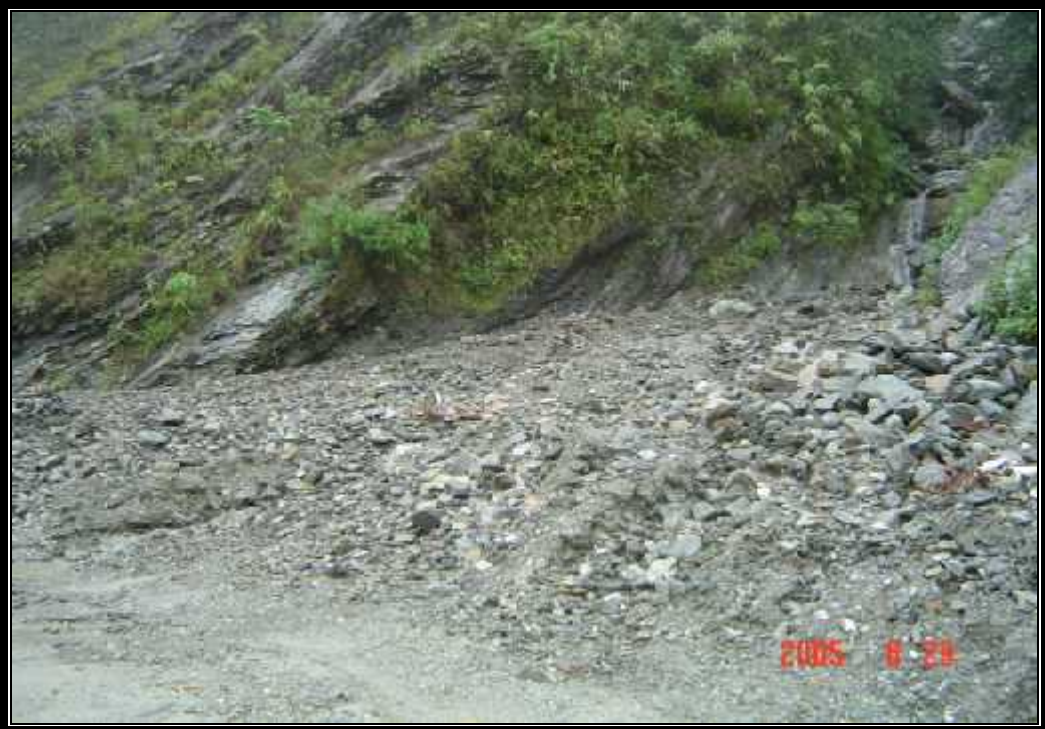
CHOKED CAUSEWAY AT NARAK JHORA SLIDE AREA, SOUTH SIKKIM
