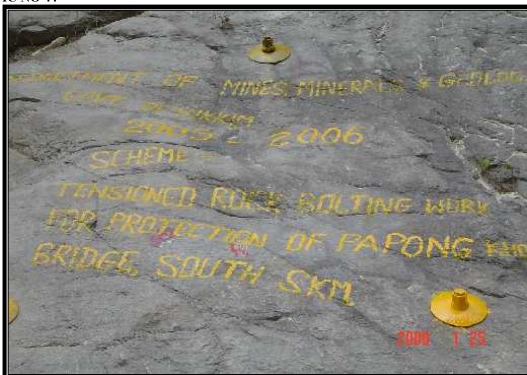
TENSIONED ROCK BOLTING BY DMM&G AT LEFT BANK OF PABONG KHOLA SOUTH SIKKIM
