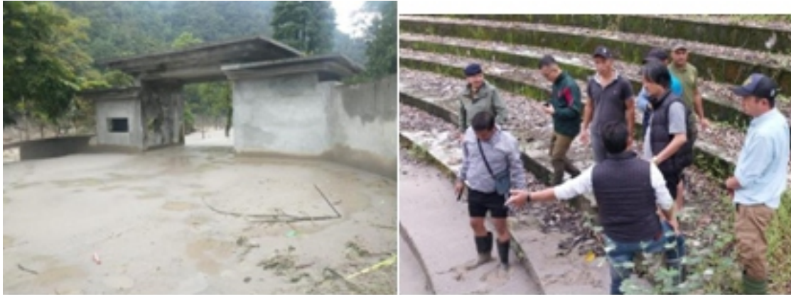
Figure 5: Representative picture depicting the damaged Biodiversity Park at Labarbotey, Dikchu- Mangan
