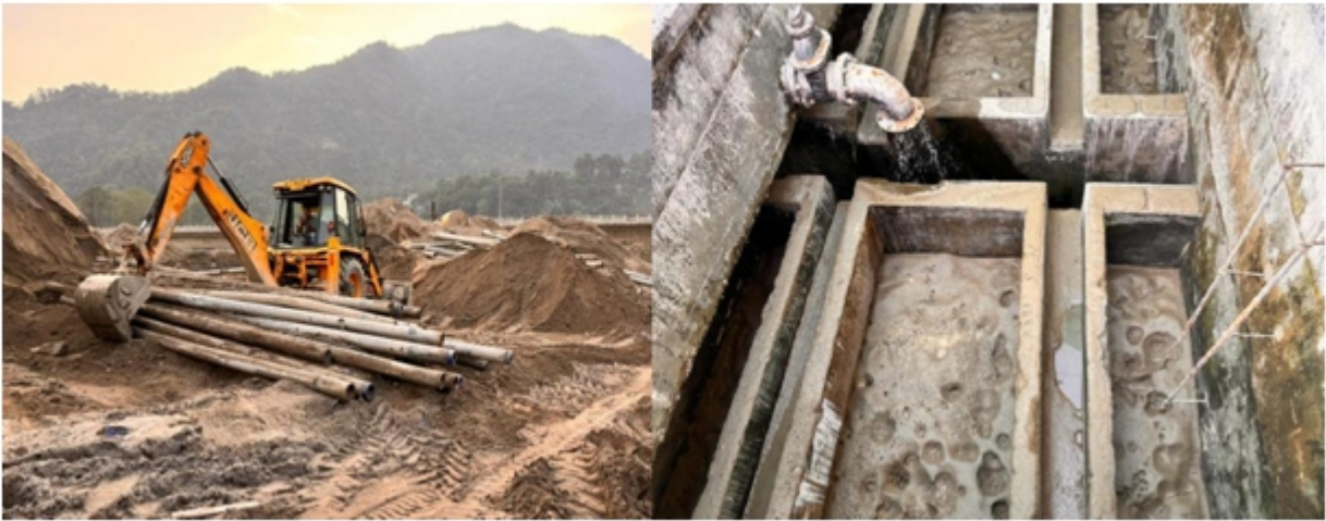
Fig: Pipes being excavated from silt IBM(left) WTP Singtam ( right) (8/12/2023)
