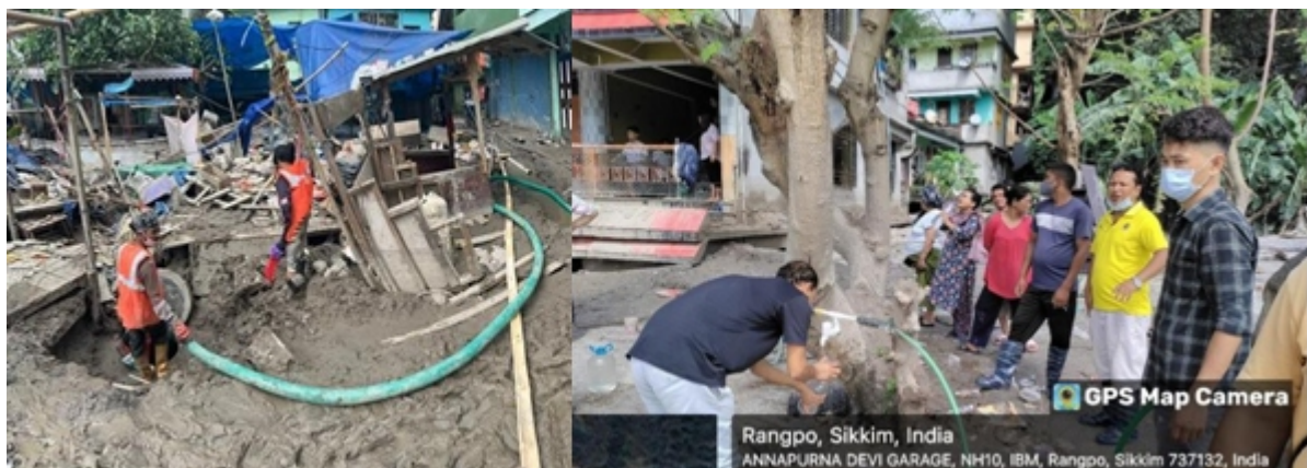
Picture: 8 sewer chamber cleaning Lalbazar, water supply Rangpo
